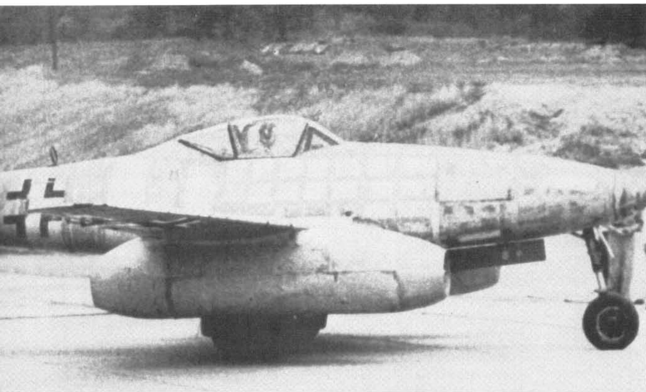
The fuselage was of semi-monocoque construction. The "checks" which appear here are the seams which had been taped and filled, but not overpainted.
