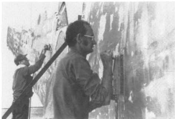
The surface was filled with body putty and sanded again.
